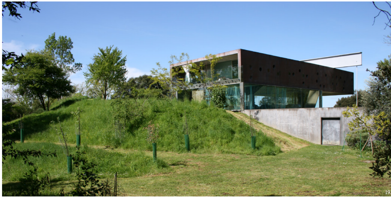
19 — Exterior back-facing view of the Maison à Bordeaux, designed by Rem Koolhaas/OMA. Courtesy of Bêka & Lemoine
